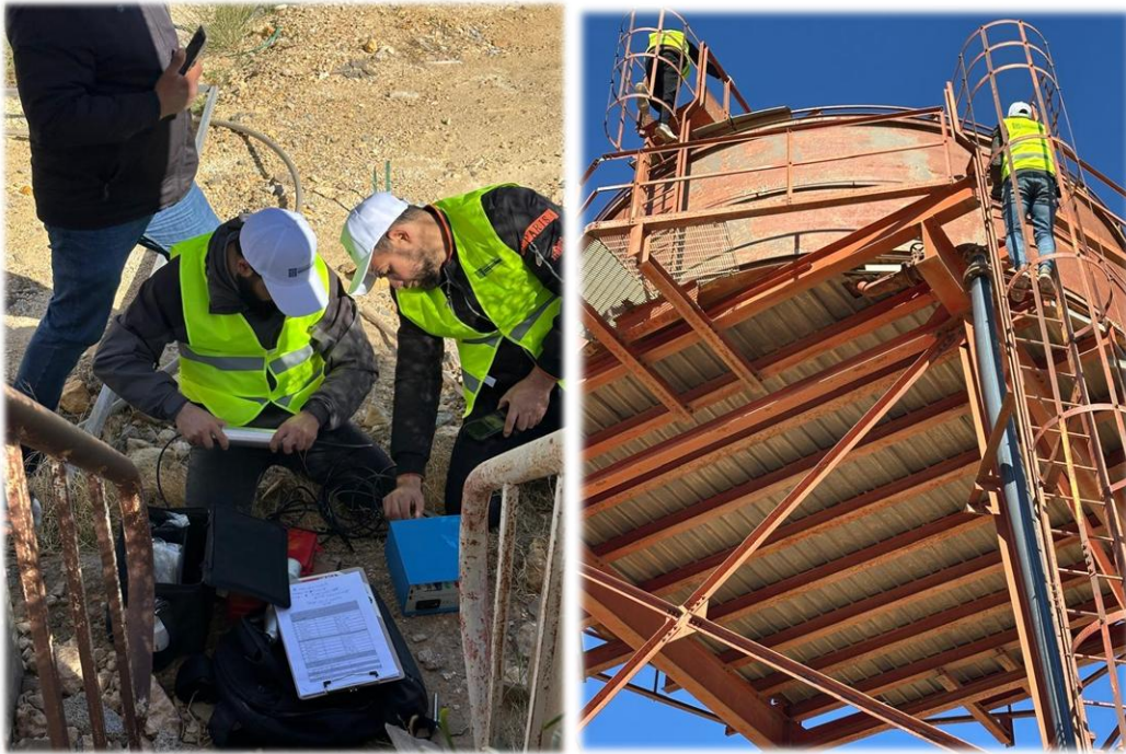
Photos 3 and 6 – Priority interventions in design and rehabilitation of critical water infrastructure © UNDP
